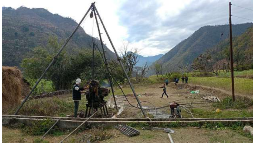
Figure 15 Drilling Process of BH-03 at Achham Site
